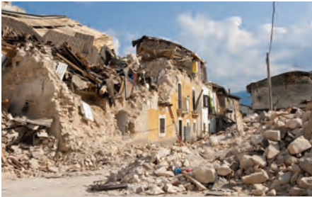
Natural Disasters; Wildfires; Landslides; CBRE incidents
